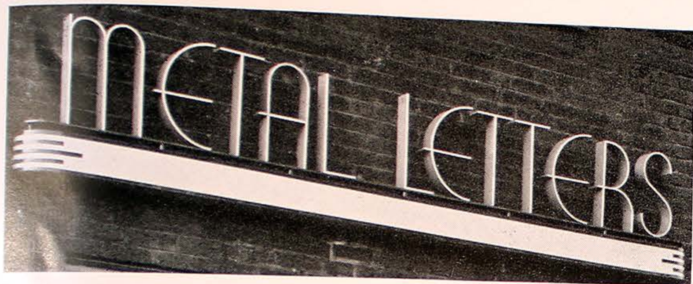
Special ribbon type letters on the Spanjer Building. Letters are 15" high, formed from 1/4x3" aluminum bar stock.
