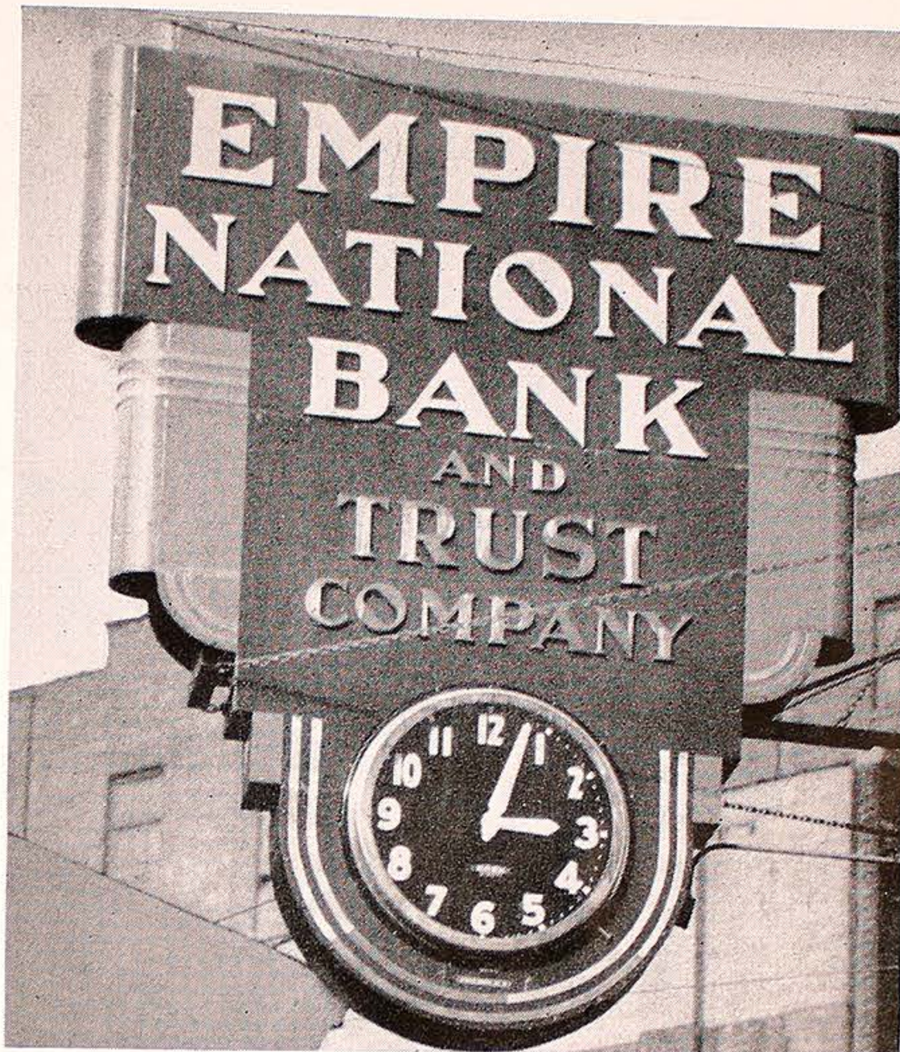
Empire National Bank letters on this large stick-out sign are made of cast aluminum; balance are bronze.
