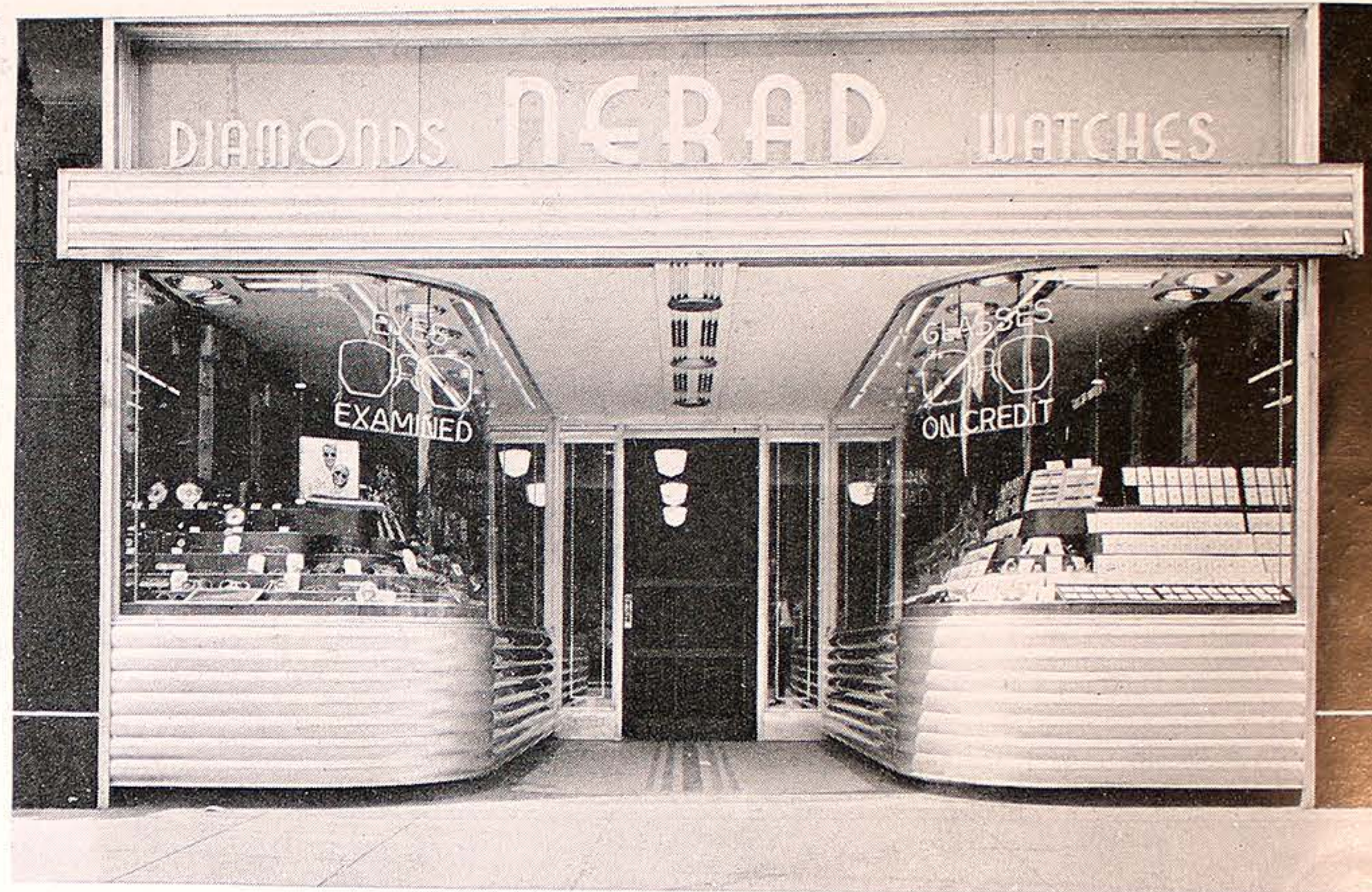
Alumilite aluminum letters 15" and 6" high mounted to aluminum base bar for easy installation. At night, letters are silhouetted in the illuminated opal glass panel.
