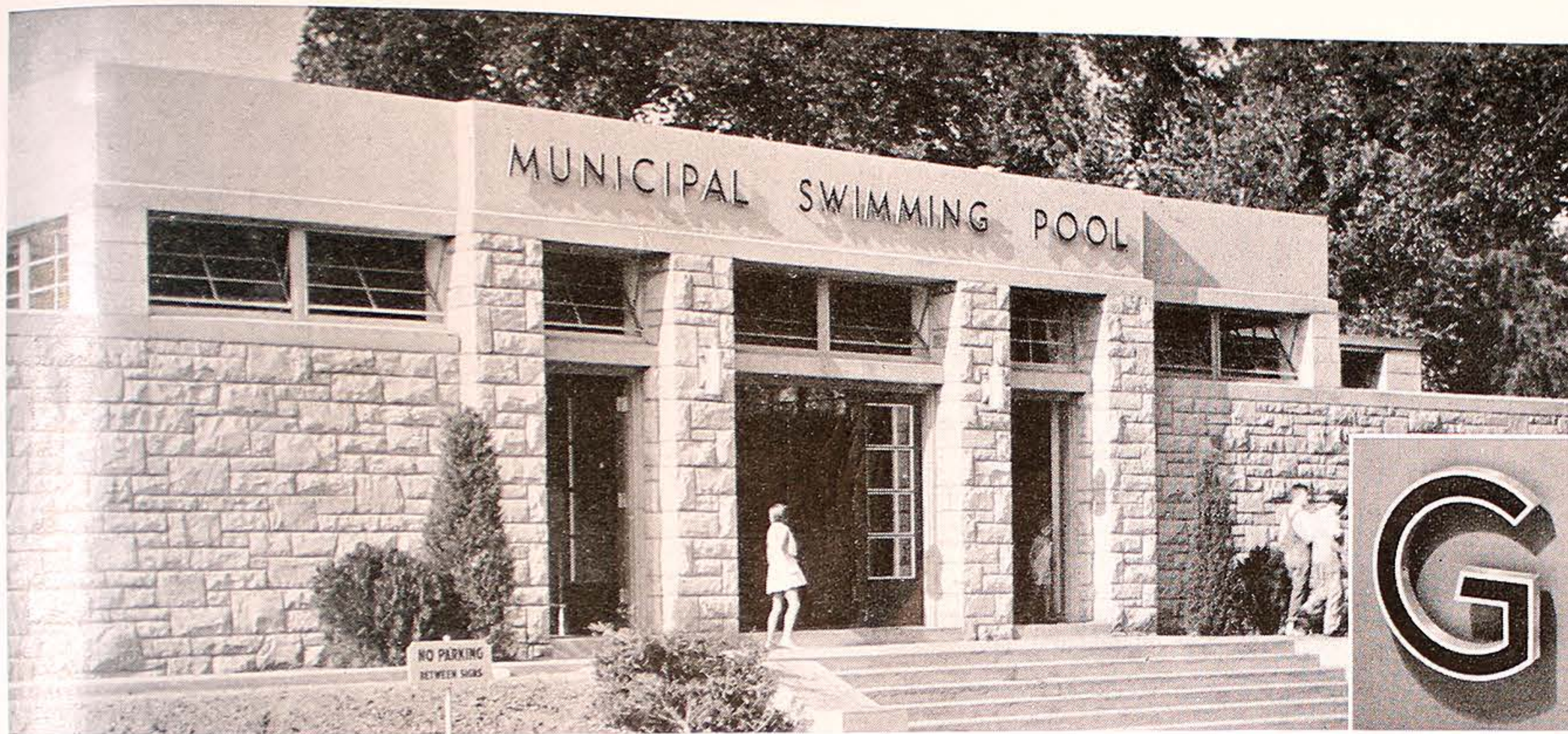
Ribbon letters, 16" high, formed from 1/4x3" aluminum bar stock, and 8" cast letters grace this modern front.
