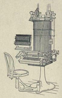
Wherever used they displace all frames and cases for body letter, except cases for the type used in correcting proofs. One machine occupies about the same floor space as a compositor's frame. In a room filled with machines twice as much type can be set as in the same room filled with frames and cases.
