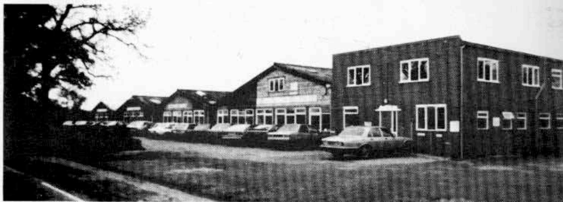
Front view of the offices and factory of D. Leonardt & Co. (Highley Pens) Ltd. 1983
